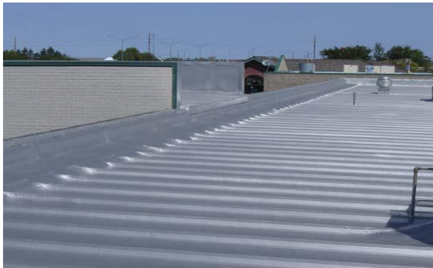
Metal Roof Coated with VFI 540 Polyurea Coating Systems
