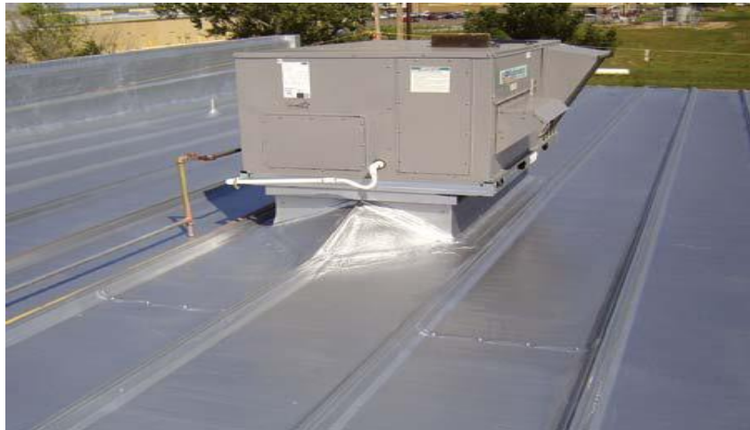
Metal Roof Coated with VFI 540 Polyurea Coating Systems
