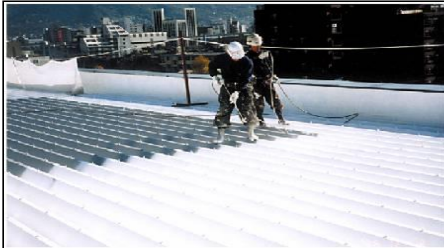
Metal Roof Coated with Ceramic Coating
