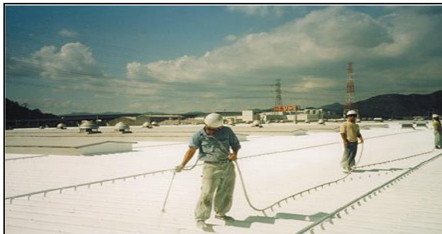
Metal Roof Coated with Ceramic Coating
