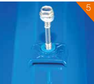
Tighten the screw to seal
